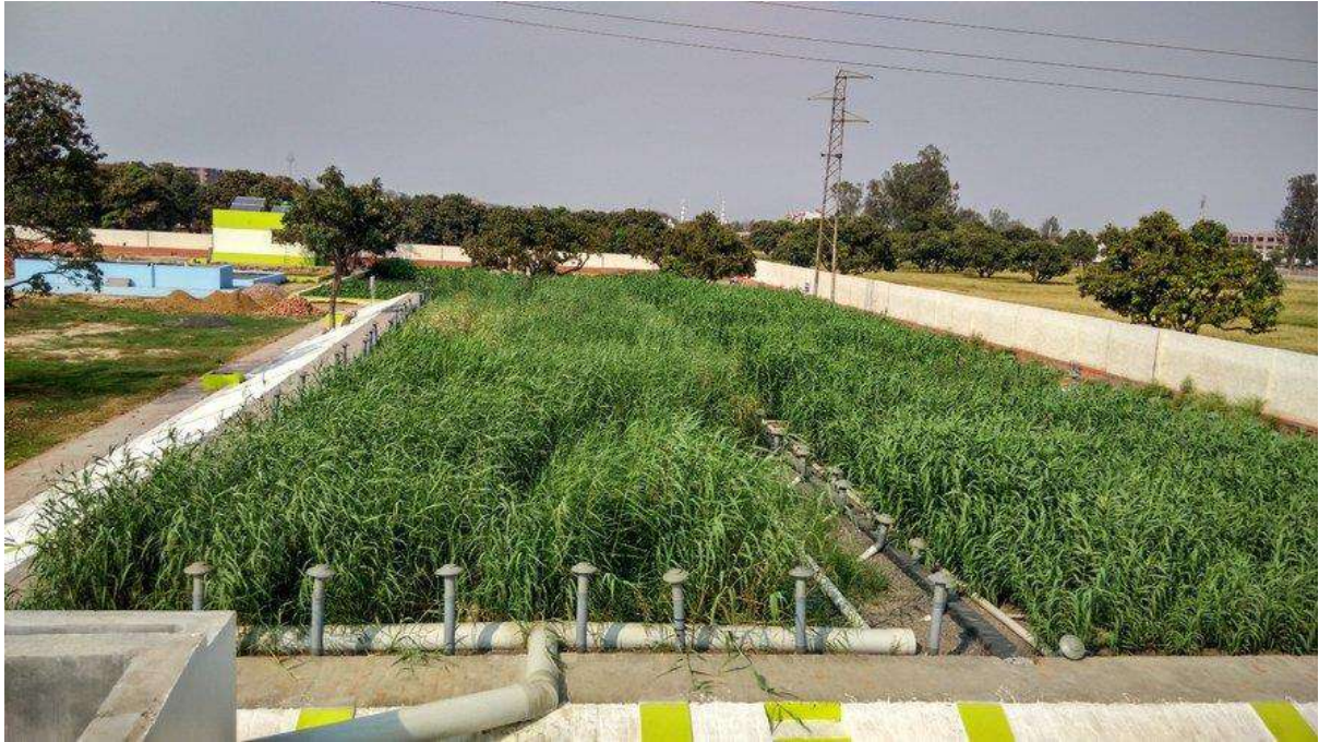
Sewage Water treatment plant
