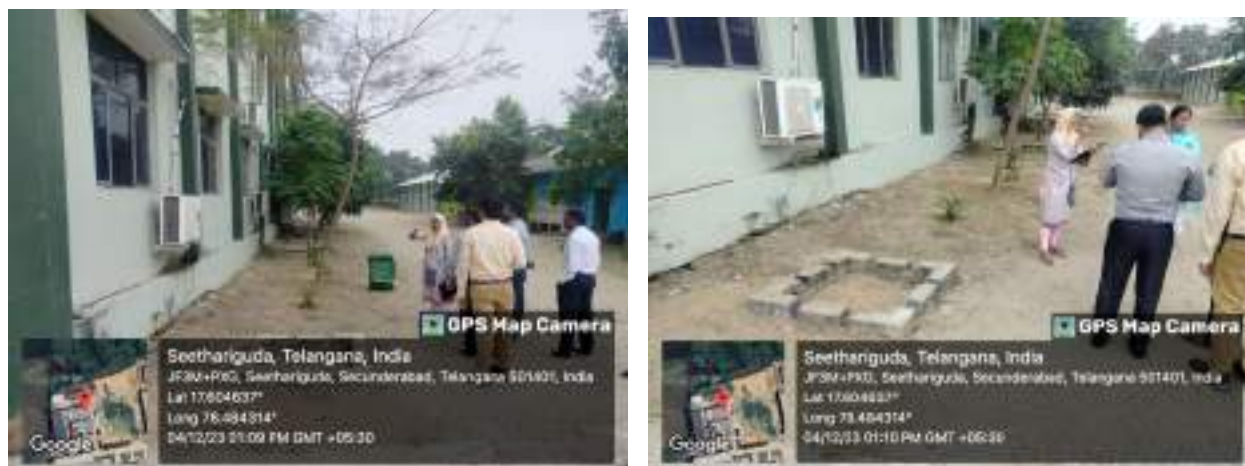
Plate 5: Rain water harvesting pits in the campus
