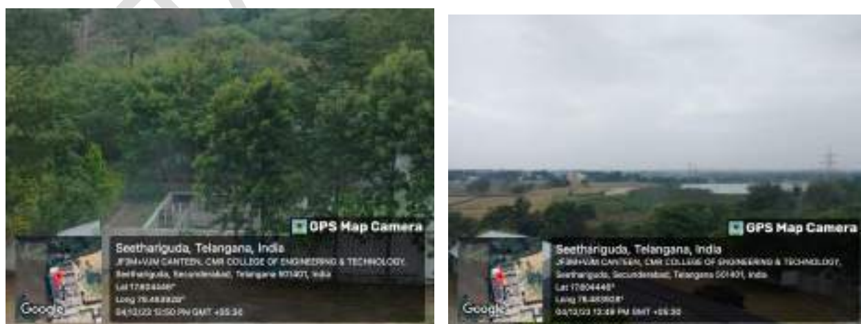
Plate 6: Sewage treatment plant and surrounding area
